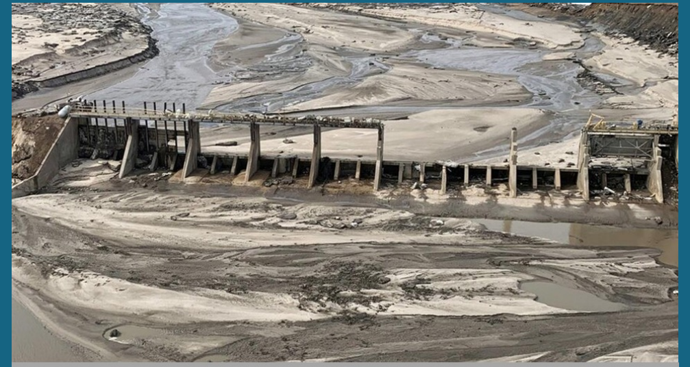
Spencer Dam; Spencer, NE; March 2019. Source: State of Nebraska.
