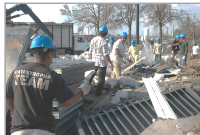
Fig. 4: Debris Removal Team
