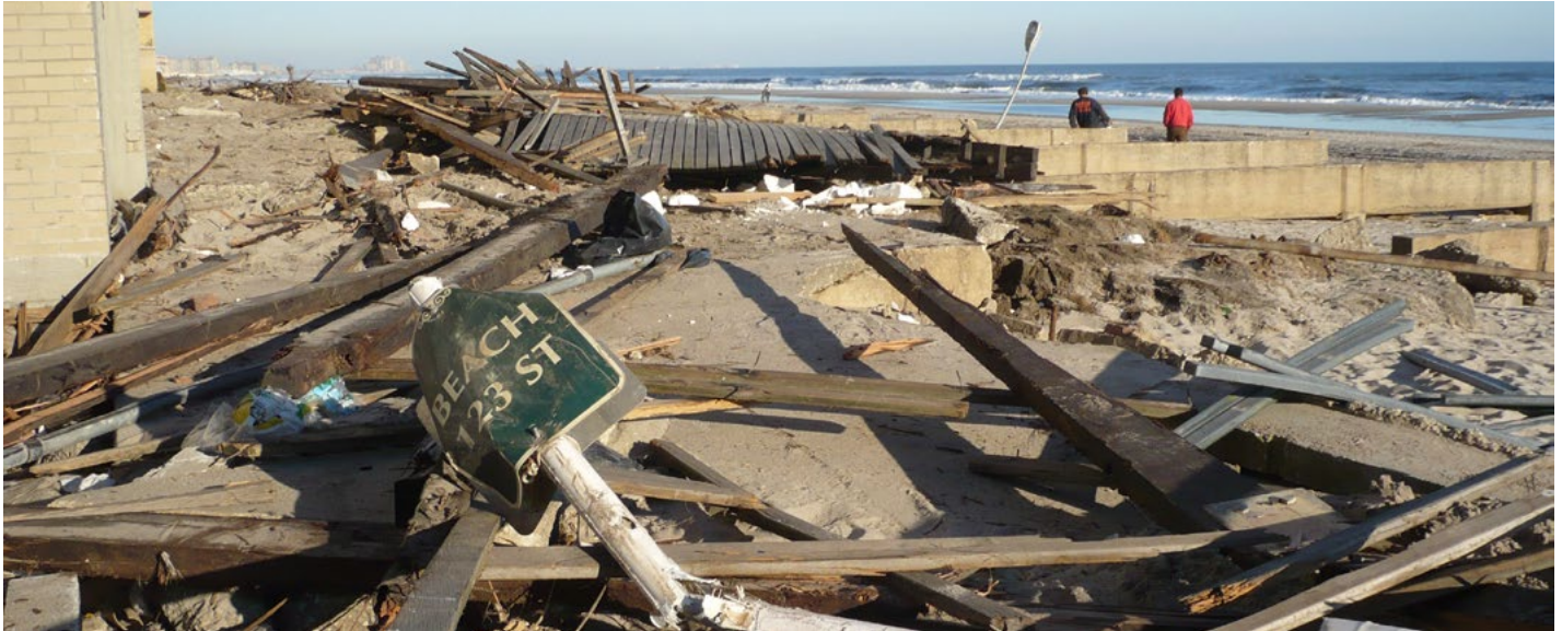
The Rockaway Peninsula was hit particularly hard during Sandy. The Governor's Office of Storm Recovery has allocated up to $21.3 million in Federal Community Development Block Grant–Disaster Recovery (CDBG-DR) monies to fund eligible recovery and resiliency projects in the Rockaway West Community. © Elke Weesjes
