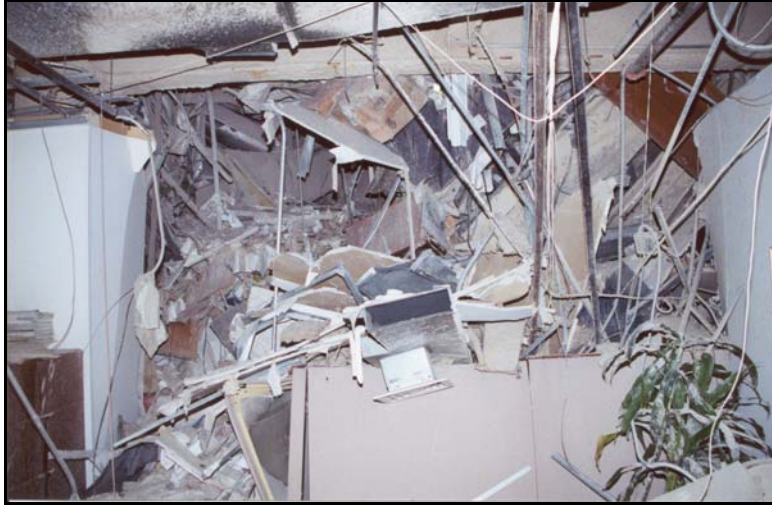
Figure 13a. Building damage at tenant level 9— complete destruction of one zone of the building.
