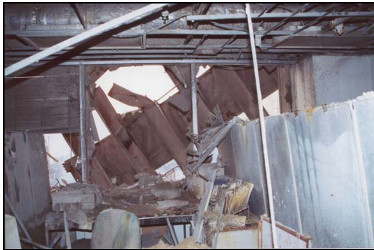
Figure 13b. Building damage at tenant level 9— view of inside face of tower 2 façade element.
