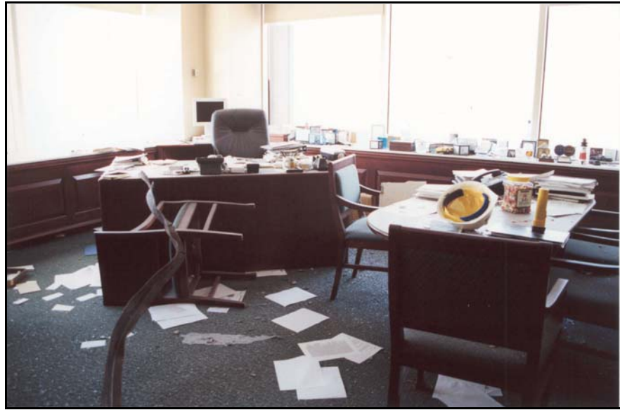
Figure 7b. Office space damage above tenant level 29— typical damage in office space.
