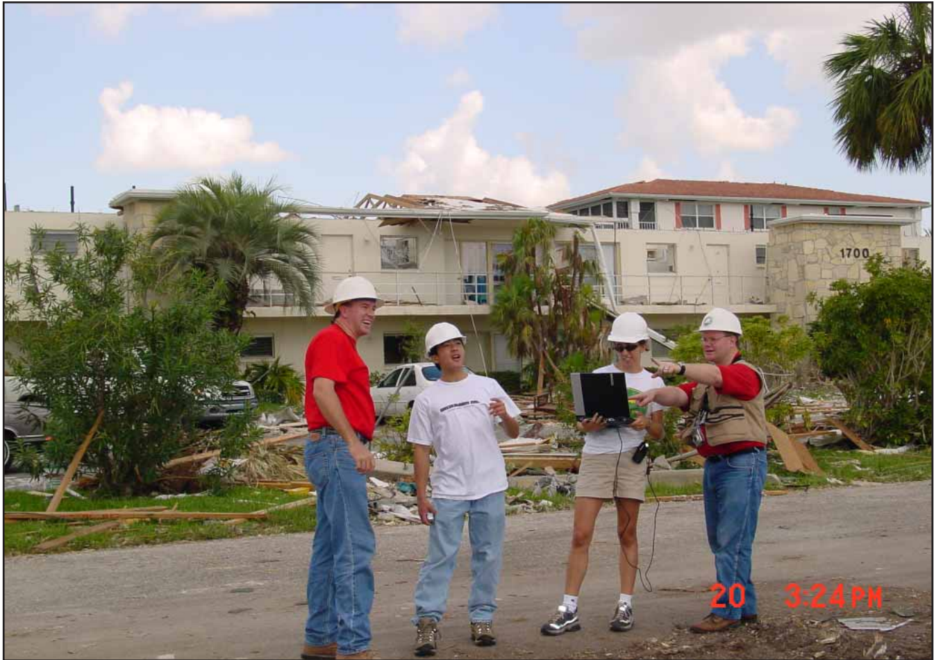
Figure 12. The field team, (from left to right) John Turner, Michael Mio, Beverley Adams and Arn Womble, outside one of the heavily damaged apartment blocks.
