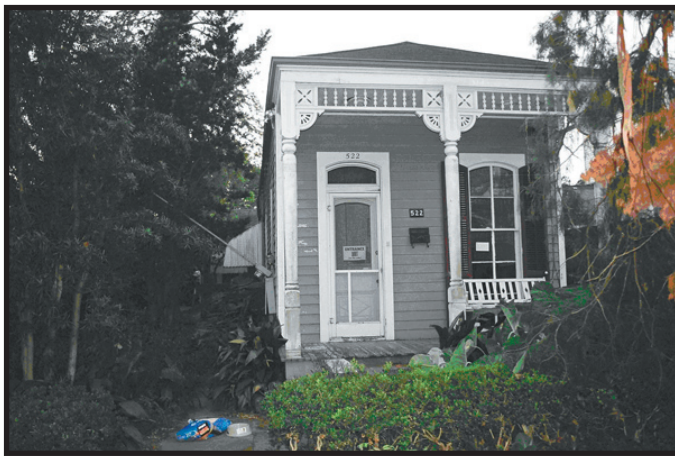
Figure 4. A damaged family home in a New Orleans neighborhood.
