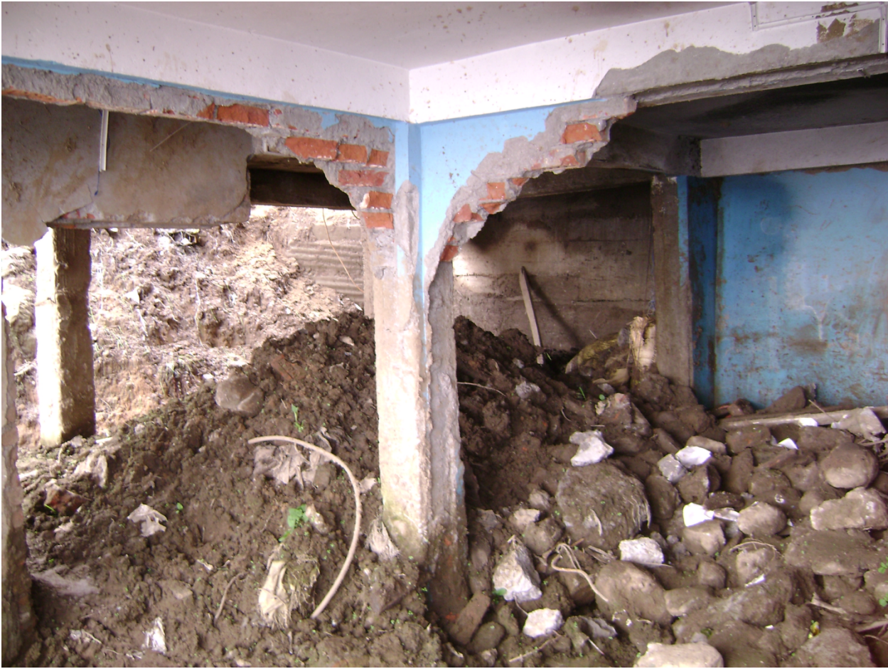
Picture 2: A house at Haridas Hatta, Darjeeling, which collapsed due to landslide following Aila killing two people
