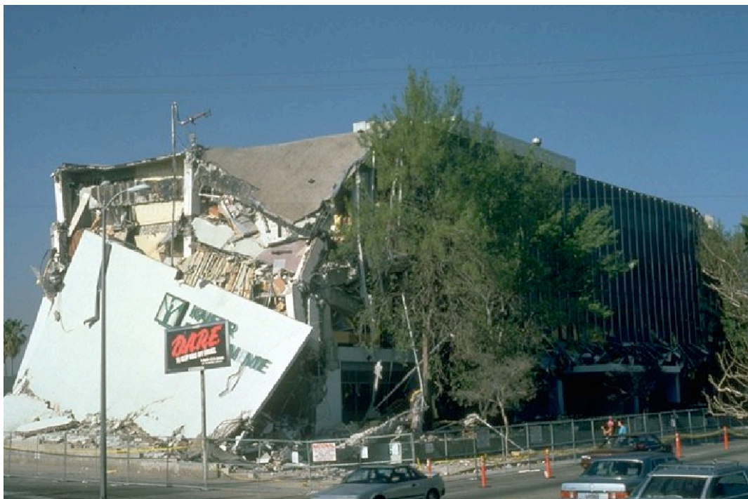
Figure 5. Overall view of Kaiser Permanente office building looking toward the northeast. The brick facades at either end of the structure have separated from the concrete frame, and the second floor of the structure has completely collapsed. The bays at the north and south ends of the building are also partially collapsed from the second to the fifth floor. Earthquake: Northridge, California earthquake, Jan. 17, 1994 Magnitude: 6.69 (Figure and caption procured from USGS archives).
