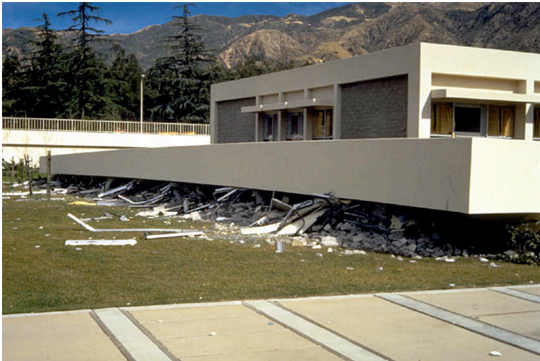
Figure 4. Olive View Hospital, Psychiatric Unit. This unit was a 2-story reinforced concrete building. The structural system was a moment resisting frame. Earthquake: San Fernando, California earthquake, Feb. 9, 1971 Magnitude: 6.6 (Figure and caption procured from USGS archives).
