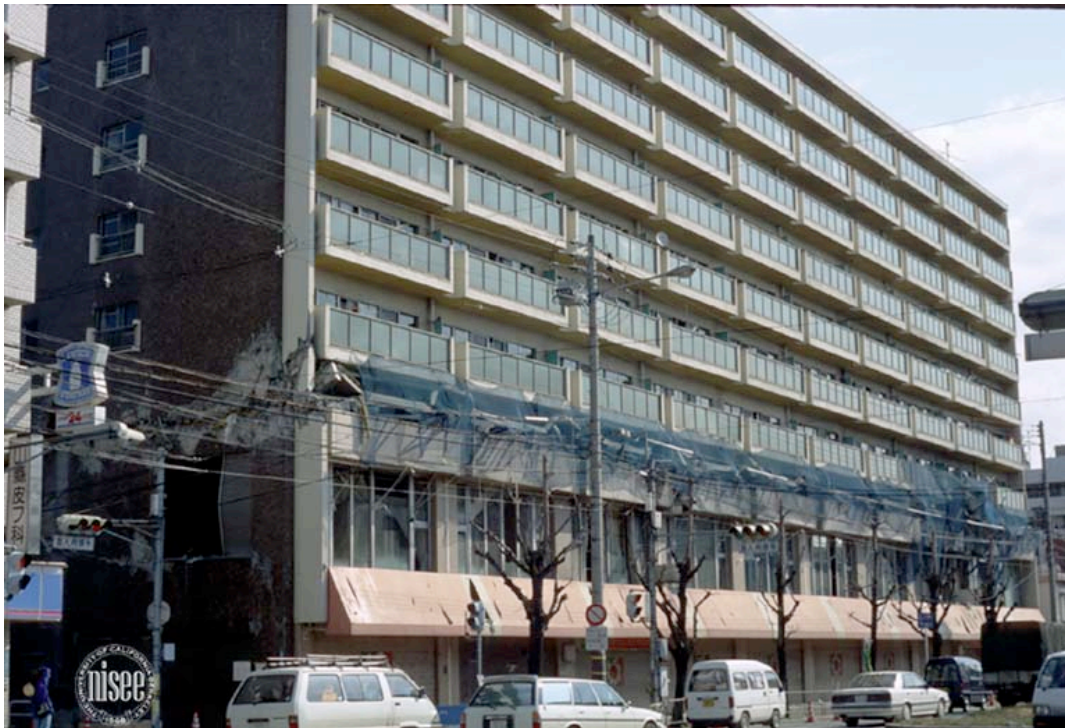
Figure 6. South elevation (front view) of an irregular, U-shaped reinforced concrete building in Nishinomiya with 3rd floor collapse. (Kobe, Japan). Earthquake: Kobe, Japan earthquake, Jan. 17, 1995 Magnitude: 6.69 (Figure and caption procured from USGS archives).
