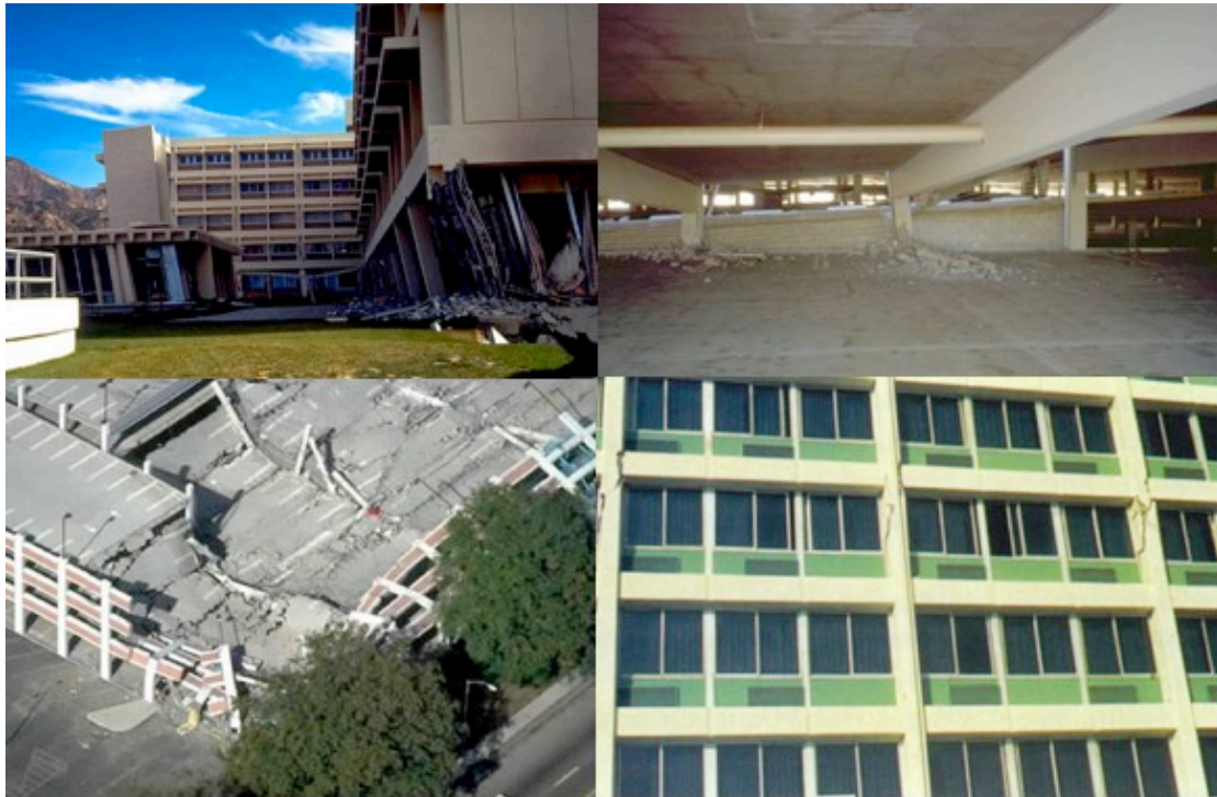
Figure 3. Damage to non-ductile reinforced concrete buildings due to 1994 Northridge Earthquake (Photos procured from USGS archives).
