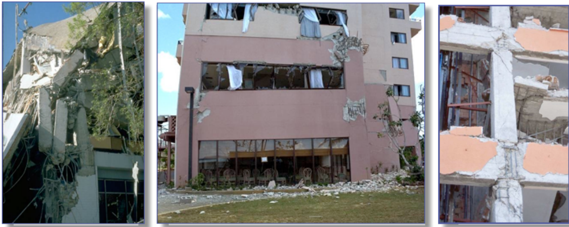
Figure 2. Joint failures observed in non-ductile reinforced concrete buildings due to strong ground shaking (Figure reprinted from Moehle et al. , 2xxx).
