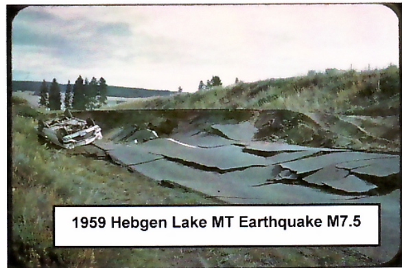
d) Damage State 5 (Total failure requiring reconstruction of pavement and underlying soils. Closure for 7 weeks)
