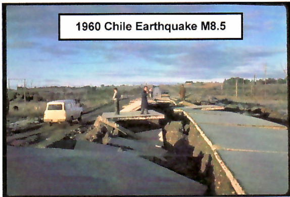
d) Damage State 5 (Total failure requiring reconstruction of pavement and underlying soils. Closure for 7 weeks)
