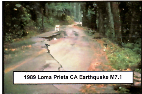
c) Damage State 4 (Pavement structure has failed and must be rebuilt, and soils have deformed. Closure for 7 days)
