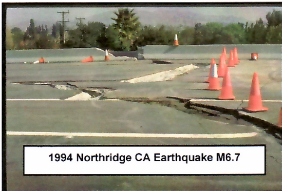
c) Damage State 4 (Pavement structure has failed and must be rebuilt, and soils have deformed. Closure for 7 days)
