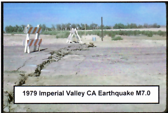
b) Damage State 3 (Closed to traffic for 2-3 days for repair of moderate pavement damage. No subbase damage)
