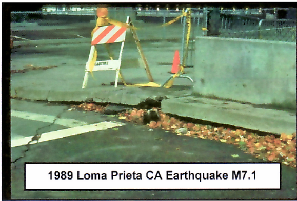
a) Damage State 2 (No closure to traffic. Minor repairs carried out during off hours)
