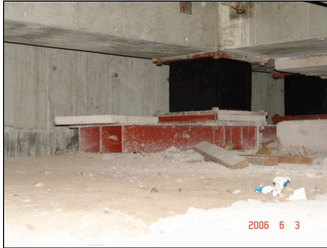
Fig. 10. Base isolator installed as a retrofit.
