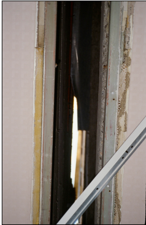
Fig. 2. Damage due to pounding at the intersection of wings of a building at Veterans Administration Medical Center, Sepulveda
