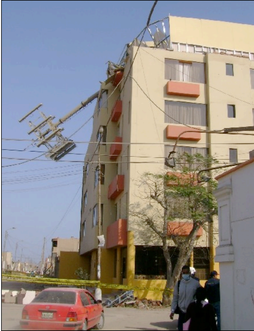
Fig. 5. Wireless phone tower collapsed.
