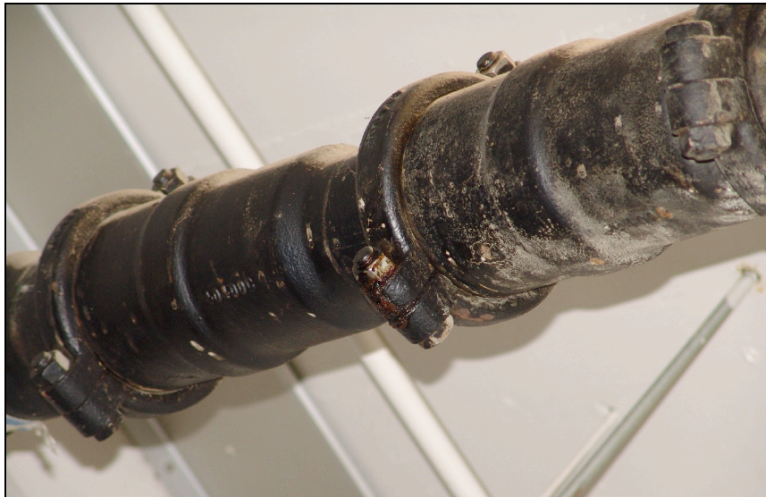
Fig. 11. Telescoping water pipe across a structural joint
