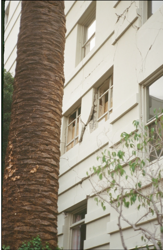
Fig. 1. Damage in non-ductile reinforced concrete frame building at St. John's Hospital, Santa Monica
