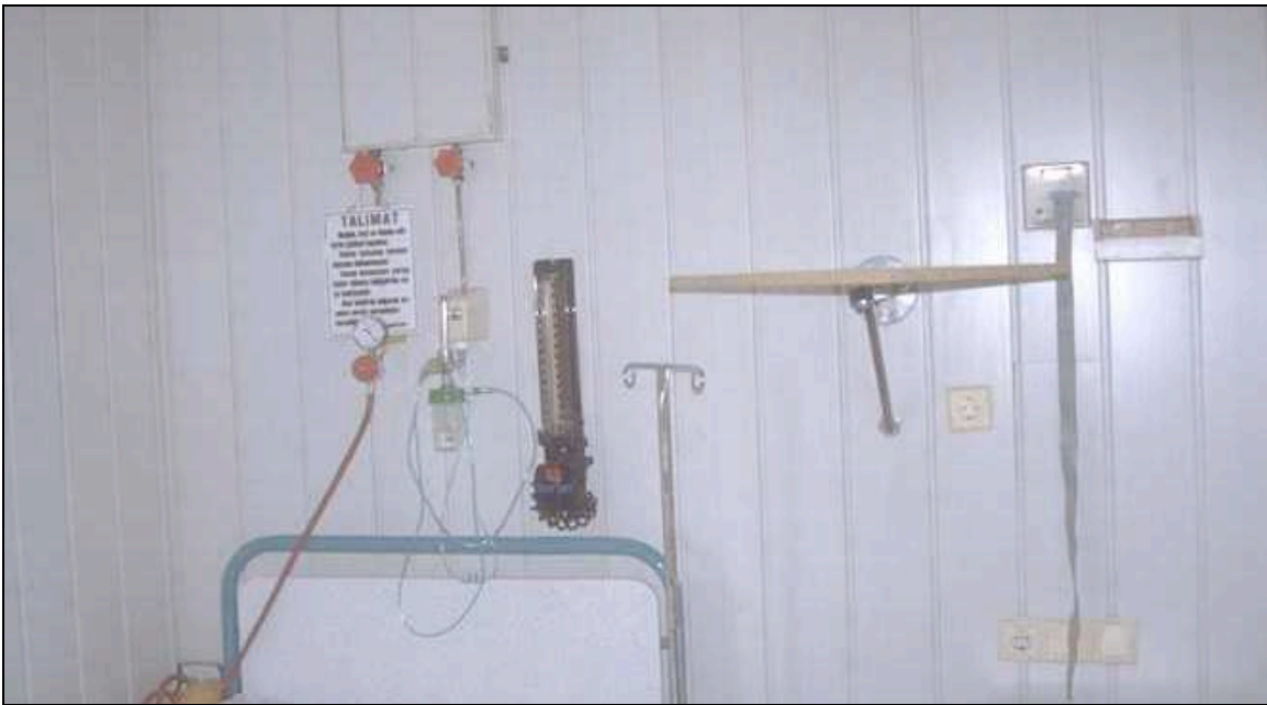
Fig. 9. Unrestrained shelf equipment fell off shelf.
