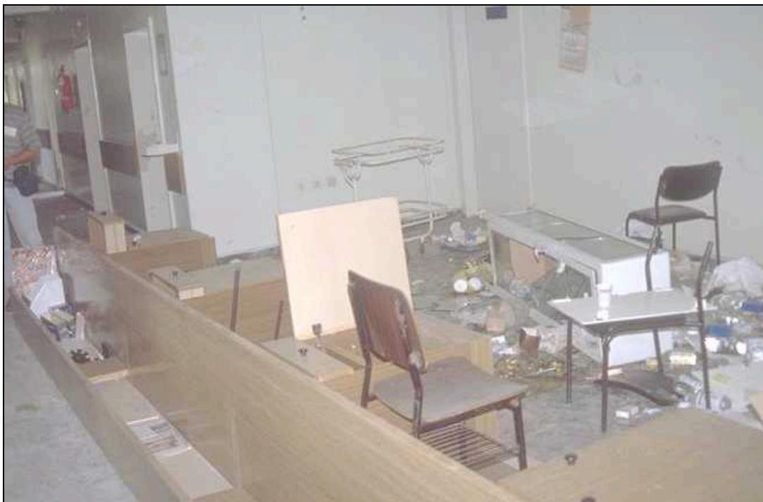
Fig. 7. Unanchored nurses' station toppled over.
