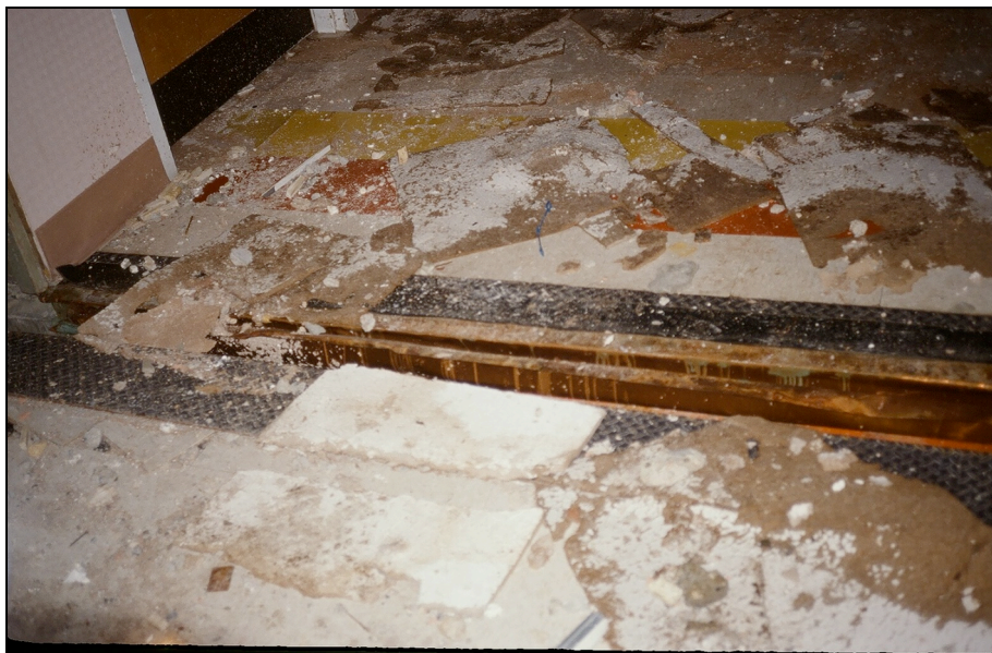
Fig. 3. Damage due to pounding at a seismic joint of a building at Veterans Administration Medical Center, Sepulveda
