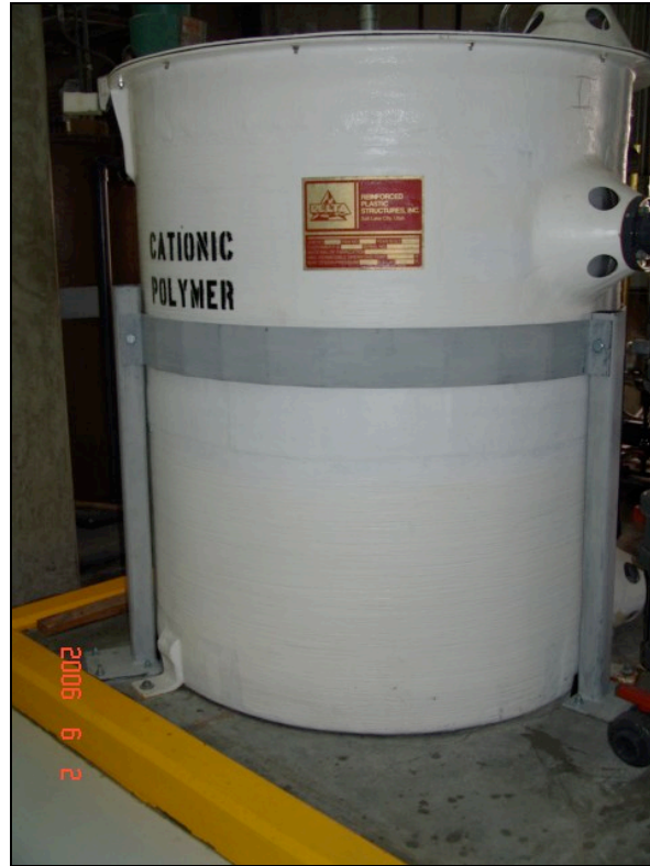
Fig. 12. Restraining anchor bolts and straps on a tank
