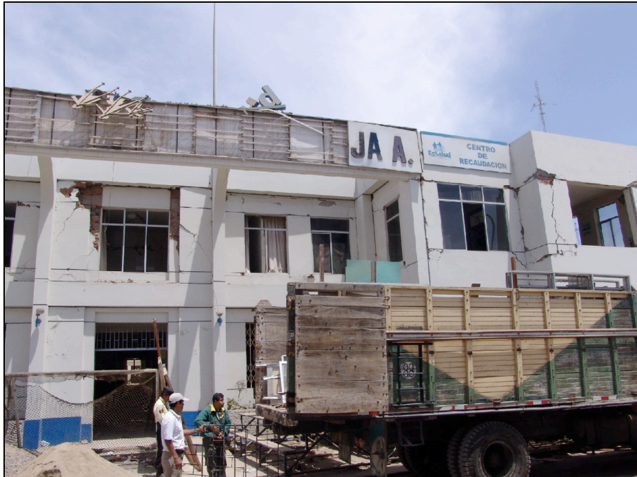
Fig. 4. Significant structural damage and loss of functionality in an unreinforced masonry hospital building, Pisco, Peru
