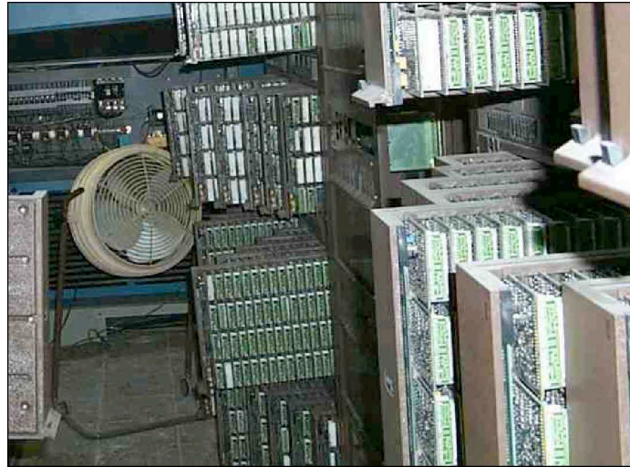
Fig. 13 Fan was used to cool the electronics, note that the units were pulled out to have better cooling effect.
