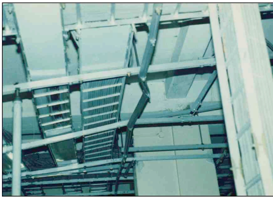
Fig. 14 The cable racks fell and were supported by jiffy poles, in Whittier Narrow earthquake.
