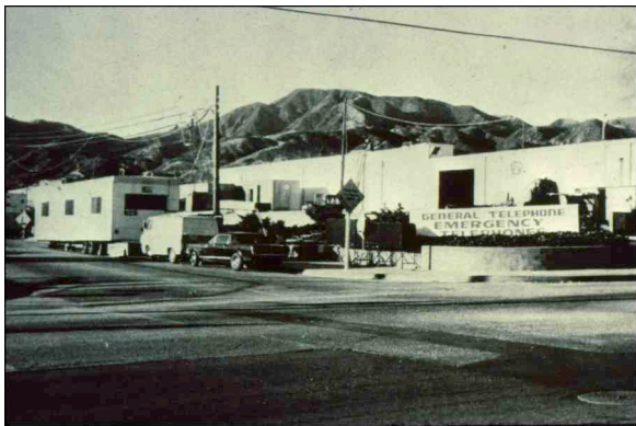
Fig. 20 This is the exterior of the CO after the 1971 San Fernando earthquake. The trailer outside housed a small switching unit to provide limited service to the area.
