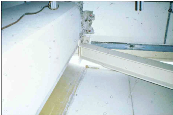
Fig. 11 This shows the anchors securing the diagonal bracing member to the structure were sheared.
