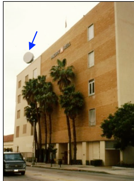
Fig. 32 Microwave dish on the roof of this CO.
