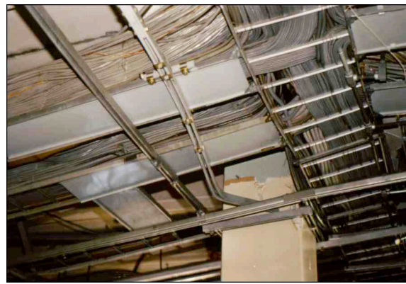
Fig. 15 This cable rack was overloaded and sustained extensive damage in Northridge earthquake.
