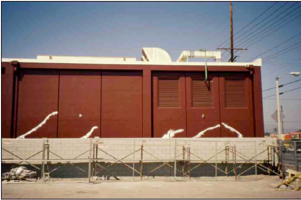
Fig. 9 A CO in Northridge after the 1994 earthquake with a few external wall cracks.
