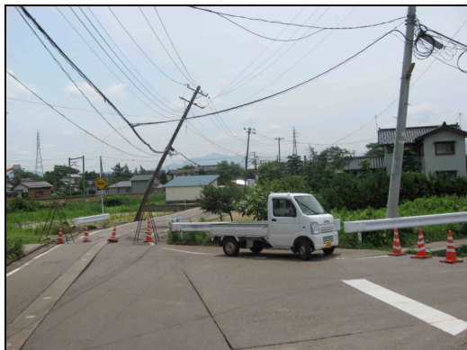
Fig. 27 Damaged poles due to lateral ground spreading
