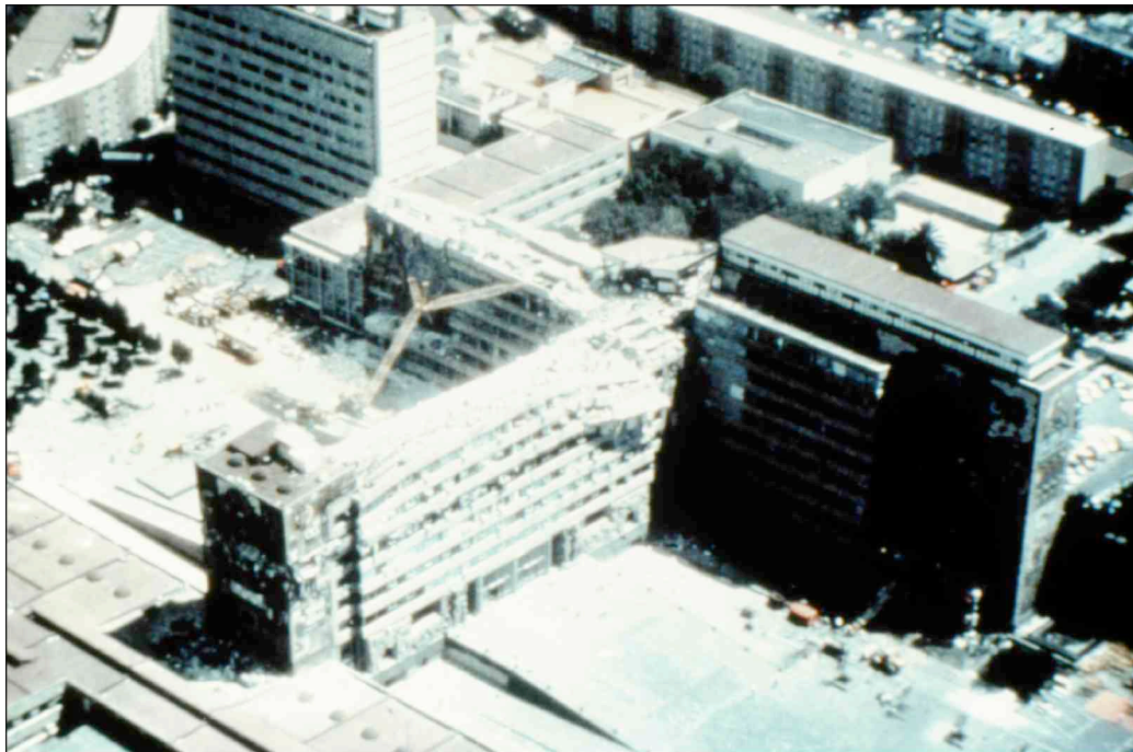
Figure 6. The top three floors of this communications building collapsed, cutting off long distance calls and significantly impacting local services in Mexico City in 1985 earthquake.
