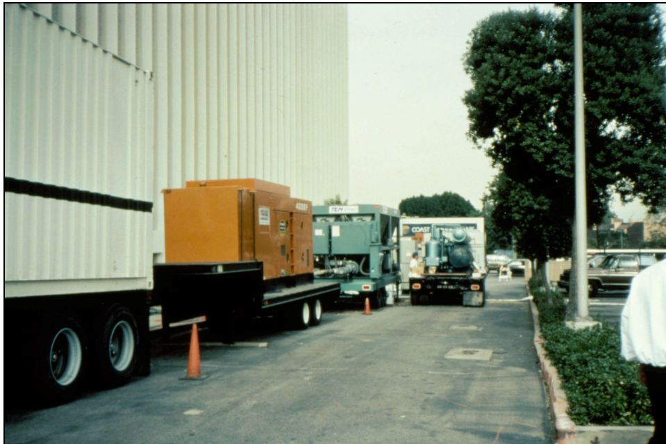
Fig. 41 Temporary mobile electric power generator was used after the Northridge earthquake at this node. The backup power generator was damaged and would be replaced. This building houses the network control center, the PSAP call center and a CO.
