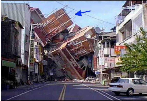
Fig. 22 A cell site that was installed on the roof of a commercial building was damaged due to building collapse. This is 1999 Chi Chi earthquake.
