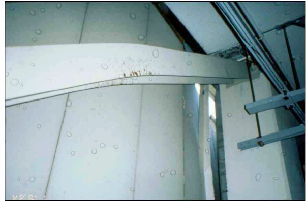
Fig. 10 This CO was upgraded, but the added bracing sustained damage but the building was saved.
