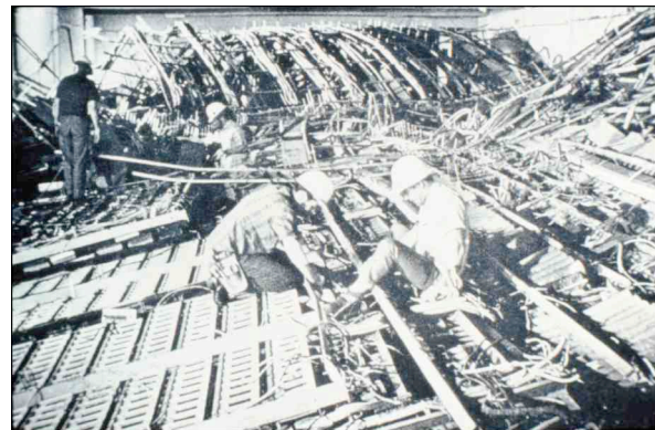
Fig. 21 The inside of the CO with all the switching equipment toppled. This was the old electro-mechanical switching unit.
