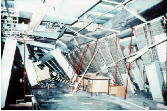
Fig. 18 This CO was non-functional equipment damage. Also this becomes a safety concern for the technicians working among the equipment.
