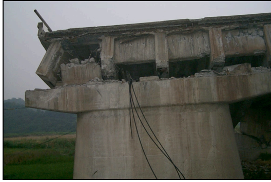
Fig. 29 One of the bridge deck collapsed and severed the cables under the bridge deck.
