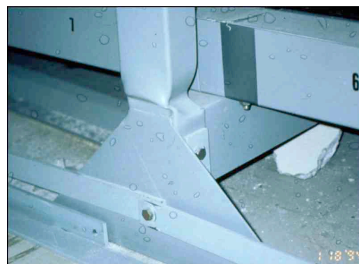
Fig. 17 This battery rack column showed insufficient load carrying capacity in Northridge earthquake.
