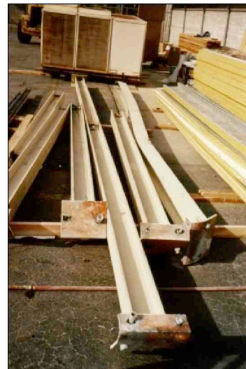
Fig. 12 The damaged bracing beams were removed and placed in the yard.
