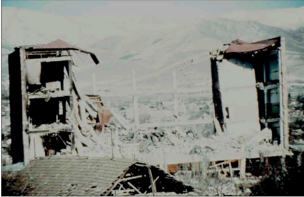
Figure 8. This Central Office in Spitak collapsed.
