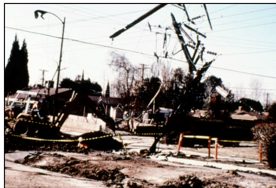
Fig. 28 Fire burned these poles taking out both electric power and telecommunications.
