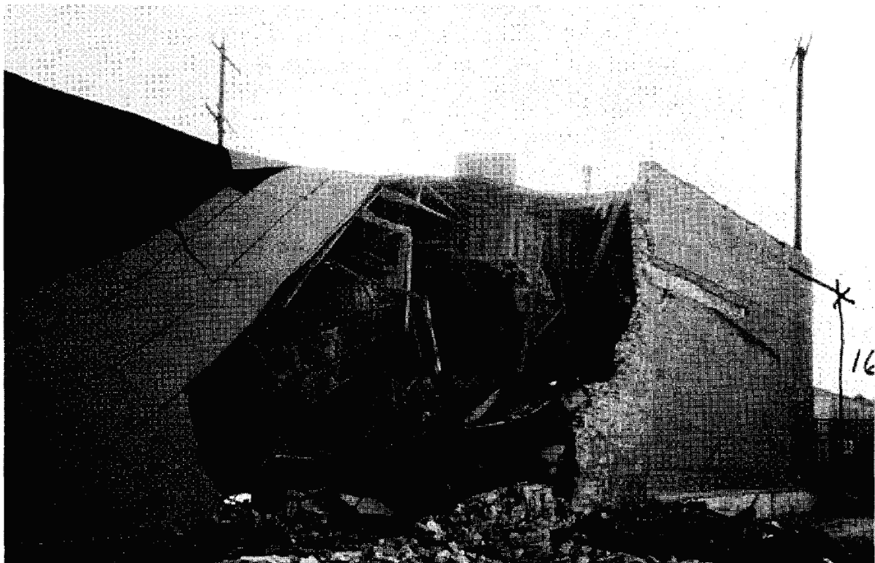
Figure 3 Partial collapse of a retrofitted URM with walls that exceed h/t limitations. (Earthquake Spectra, January 1996 Supplement C to Volume 11)
