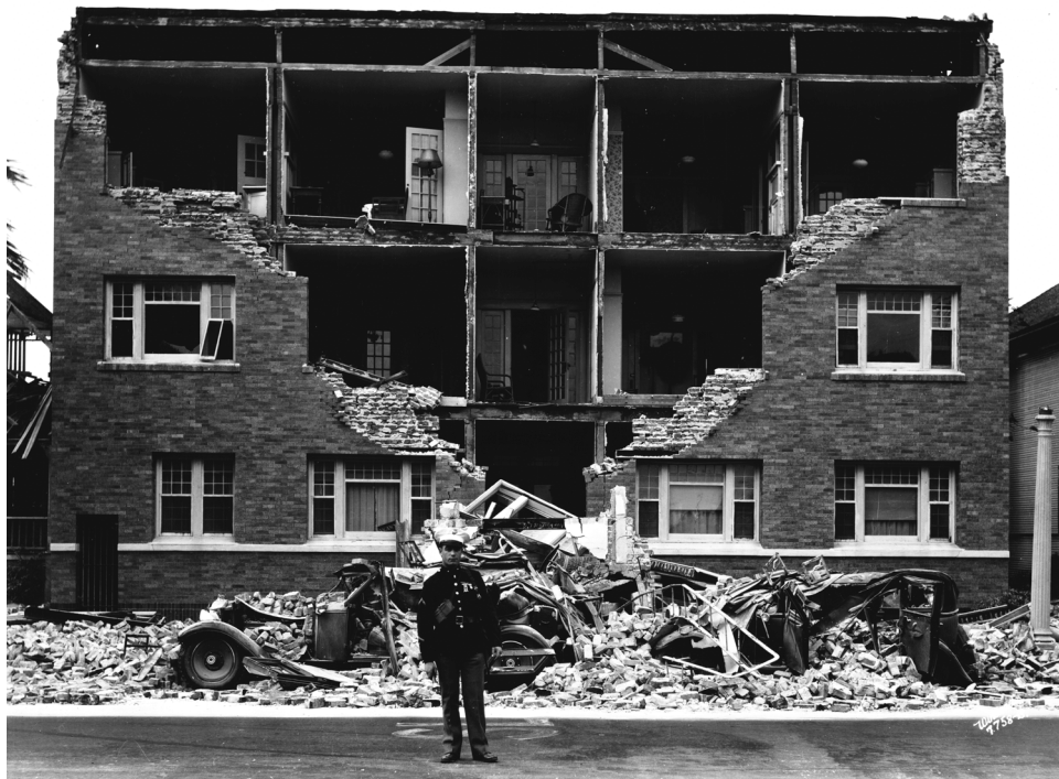
Figure 2 Morrison Apartments, 915 E. Ocean, Long Beach, California 1933 – Front wall only fell away from floors and roof onto street below due to directional properties of earthquake (Historical Society of Long Beach, PO Box 1869, Long Beach, CA 90801 (562) 424-2220)
