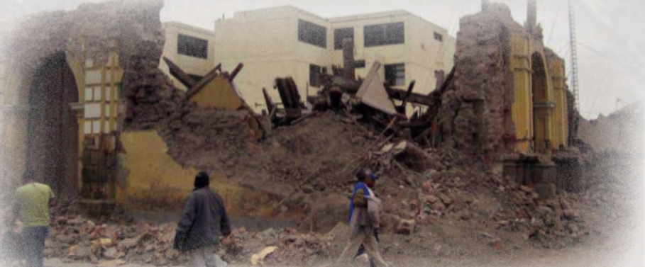
Collapsed adobe church in Pisco, Peru, following the August 15, 2007, magnitude 8.0 earthquake. For events such as this, PAGER provides emergency relief organizations with information that helps them determine which areas likely require the most attention. Photograph by Emily So, EEFIT, United Kingdom.
