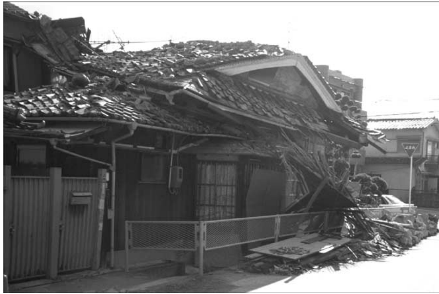
Photograph 2. Example of possible building assessed by visual inspection from outside.
