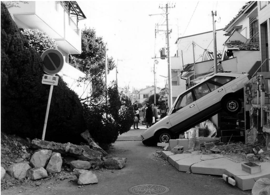
Figure 4. Earthquake damage in Kobe. (Photo: Robert B. Olshansky)
