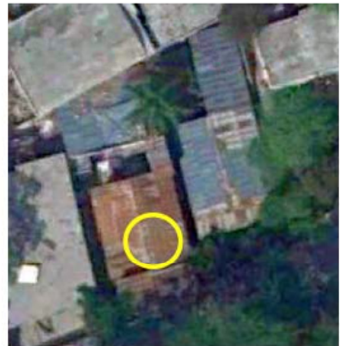
No visible damage: Assessed building does not appear to be damaged. Here: Centre building with brown roof seems intact. No debris or collapsed structure is observed. Neighboring buildings do not show damage either, providing contextual information to help decide on the "no damage" state.
