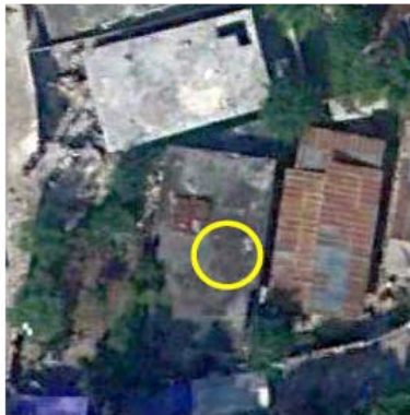
Level 3 - Substantial to heavy damage: Limited damage observed to building, or no damage observed but immediately adjacent to destroyed or very heavily damaged building. Here: Centre building assessed has limited damage (some debris to the left of building), but bright building adjacent (above) severely damaged as seen in collapsed walls (debris to the left of building)
