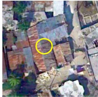
Level 4 - Very heavy damage: Part of building structure collapsed, such as part of roof or one or more fallen walls. Wall fallen into street (bright debris)
