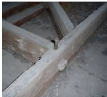
< Fig. 23. Attic framing with mortise and tenon joinery with wooden peg.
