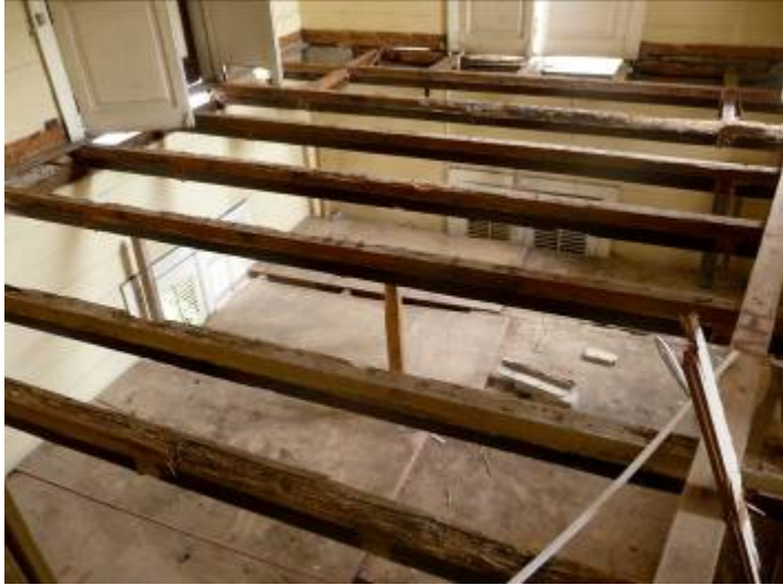
Fig. 19. Wood floor framing with wood plank floor removed. (32 Lamartiniere)
