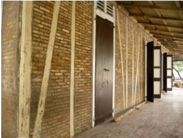
Fig. 12. Colombage with brick and lime mortar infill. (30 Lamartiniere)
