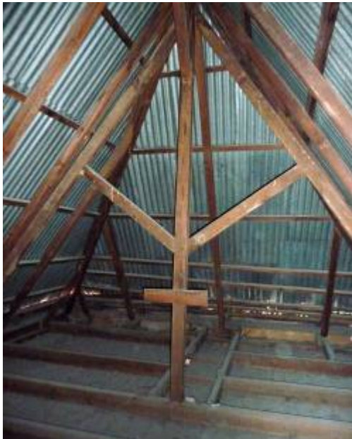
< Fig. 21. Corrugated steel roof with braced roof framing.
