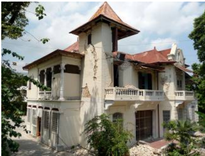
Fig. 9. Masonry bearing wall structure. Exhibits partial collapse of corner tower. (Catholic seminary, 110 Rue Fleur Du Cheine)
