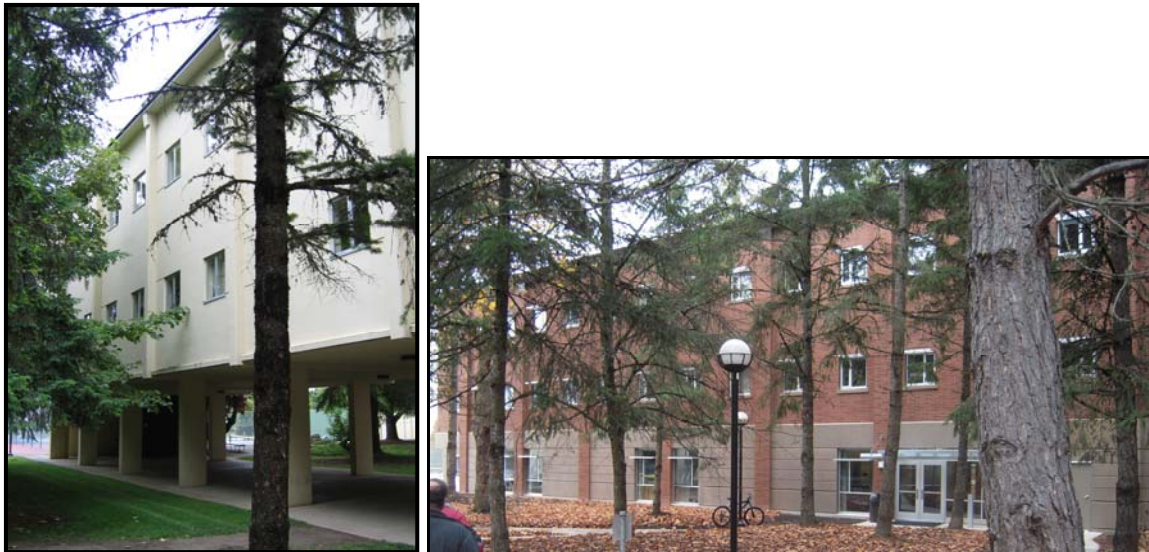
Figure 5. Before (left) and after (right) mitigation of soft-story, collapse-prone building at Western Oregon University in Monmouth, Oregon.
