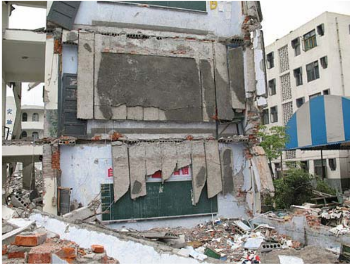
Figure 6. Damage to a school in the 2008 earthquake in China. Floor boards are hanging down on the green chalkboard. Photo: Kit Miyamoto.
