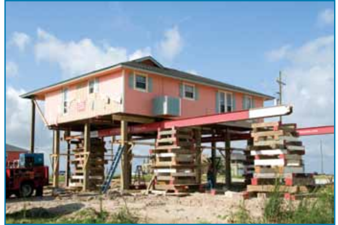
A home is elevated to comply with requirements for homes being built or repaired in Crystal Beach – May 2010.
