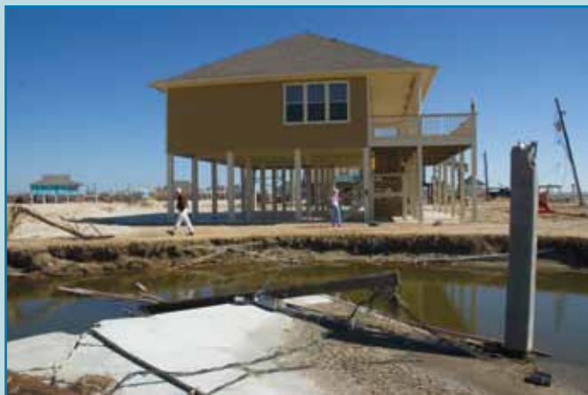
The Bishops’ house survived Hurricane Ike nearly unscathed.
