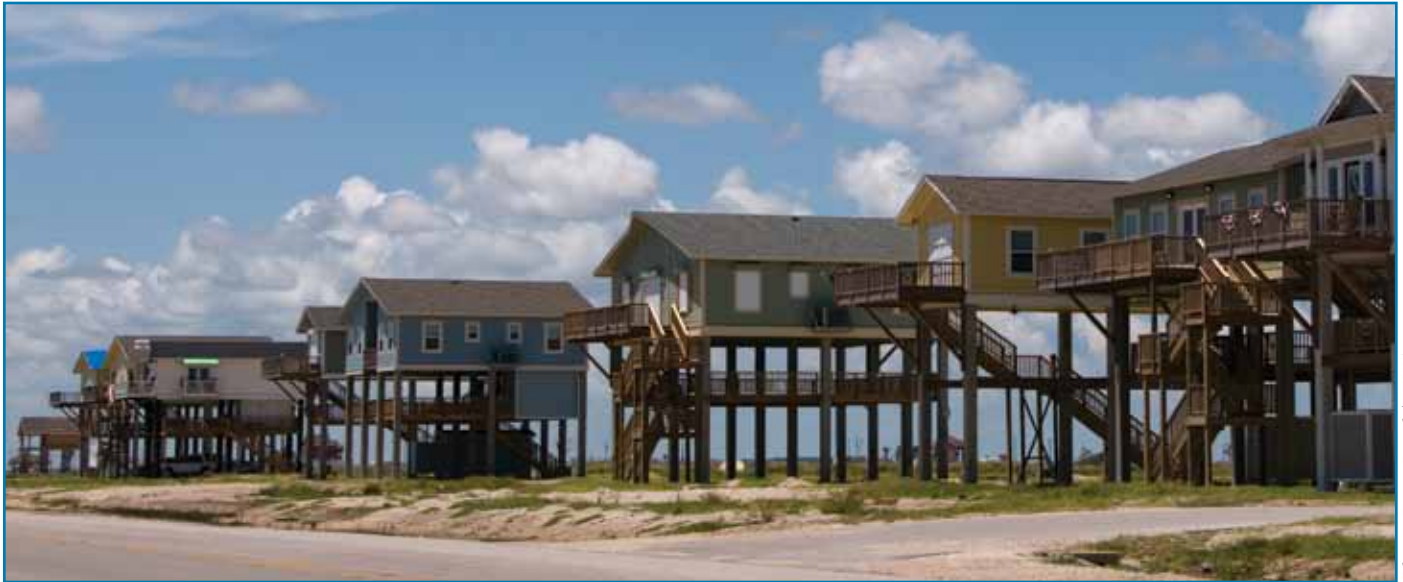
A cluster of elevated houses was damaged but survived Hurricane Ike.
