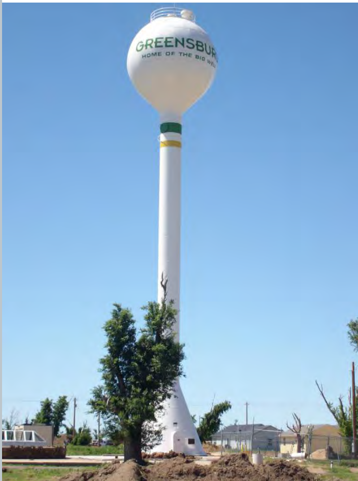
Greensburg Water Tower
