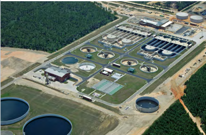
Central Water Reclamation Facility
