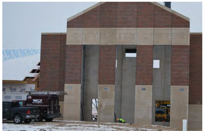
Palo City Hall/Community Center under construction
