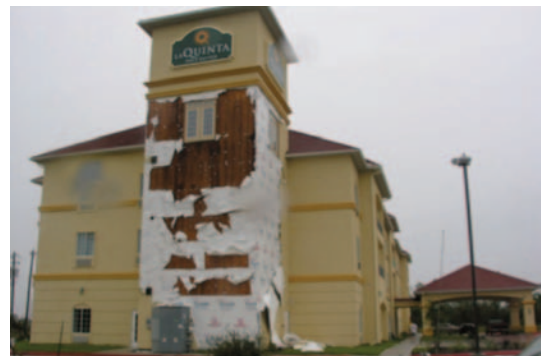
Source - Institute for Business & Home Safety
