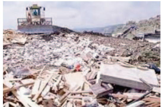
Source: U.S. Department of Energy
