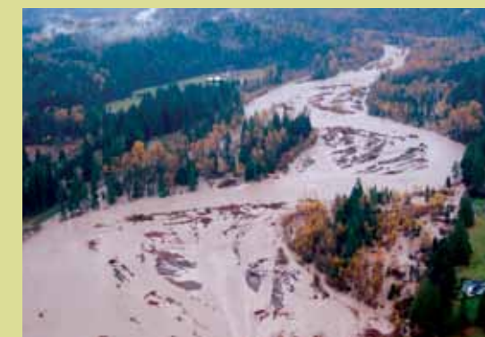
Ford Setback Levee | Photo: Pierce County Water Programs, WA
