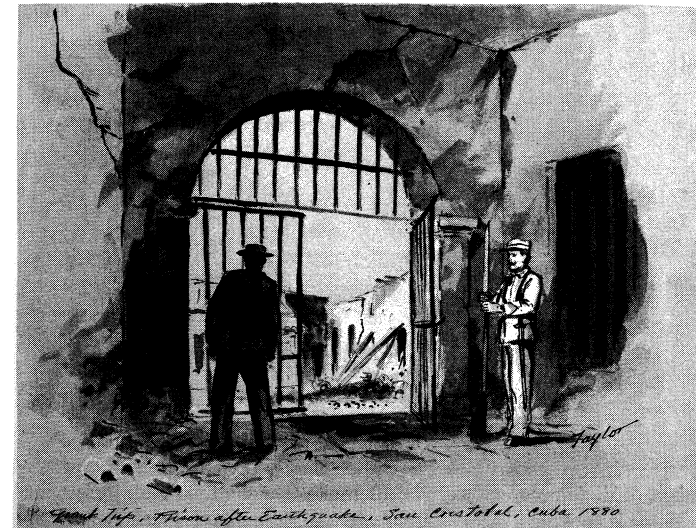
Image 4: The cracks in the walls of the mortar structure made the entire building unstable. The Prison after the Earthquake . Frank Hamilton Taylor. Sketches of Cuba, from the pamphlet "A Stately, Picturesque Dream"
