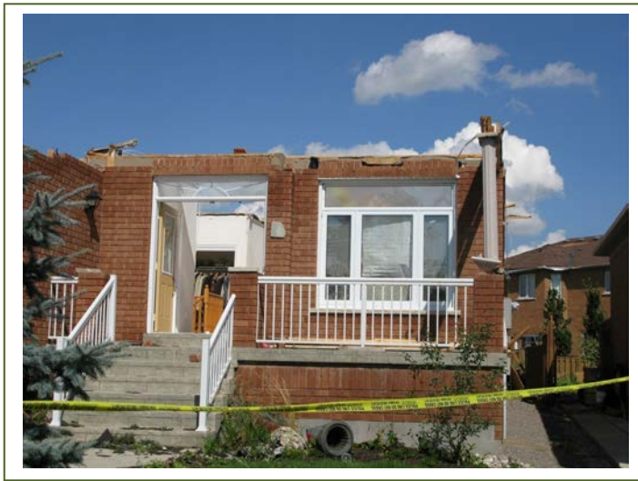
Figure 1: Two side-by-side houses, photographed the day after a tornado in southern Ontario. One lost the roof, the other only lost a handful of shingles. The difference: for the house on the left, the front doors blew in allowing the wind to pressurize the house causing the roof to fail.
