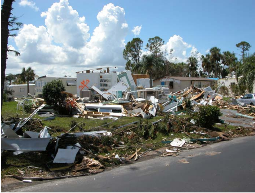
Figure 8. Differences in damage in Port Charlotte Village.
