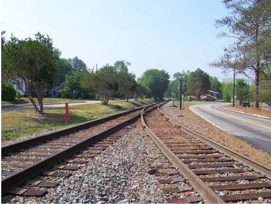
Figure 5. Graniteville derailment site: The train was to travel north through Graniteville on the main line (left track). A missed switch sent the train onto the right-hand spur and into a parked locomotive. The photo looks toward the south.
