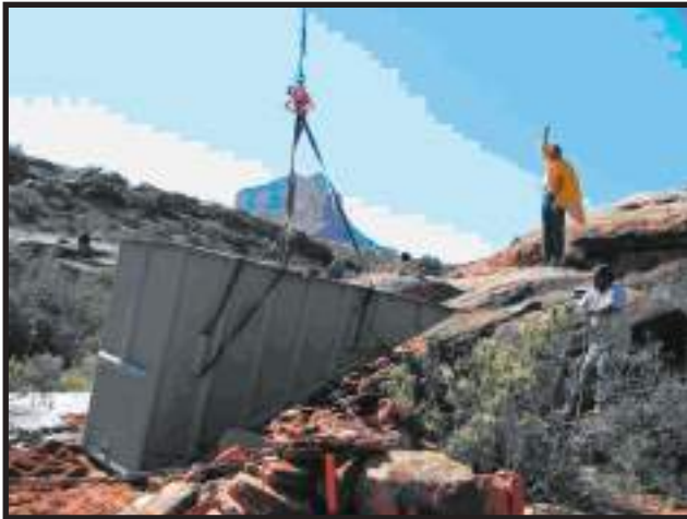
Figure 6. Installing remote wildlife “drinkers” by helicopter in 2005
