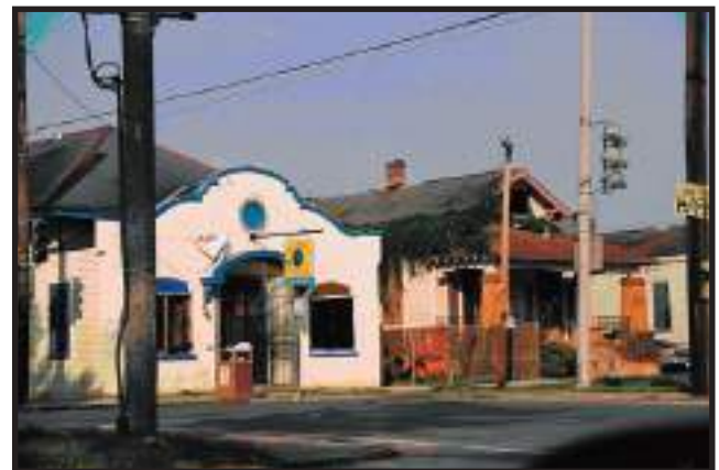
Figure 7. Kid's World, a preschool located in New Orleans, had not yet reopened following the hurricane.
