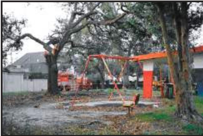
Figure 6. This children's playground, located in New Orleans, sustained heavy damage in the hurricane.
