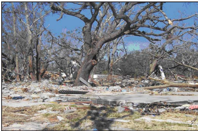
Example of house foundation pad in Mississippi. Coastal homes were often swept away, leaving only the concrete pad.
