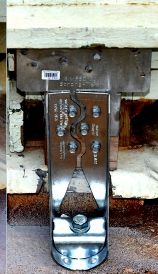
Short Holddown & Titen Concrete Anchor Screw
