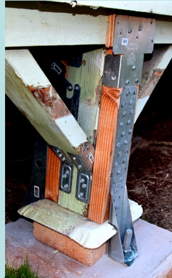
Long Holddown & Epoxy Anchor Bolt
