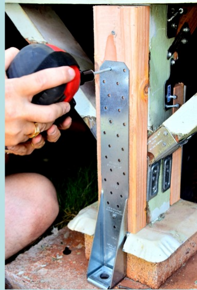
Long Holddown & Epoxy Anchor Bolt
