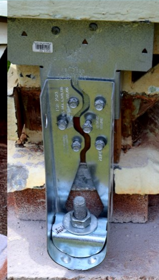
Short Holddown & Epoxy Anchor Bolt
