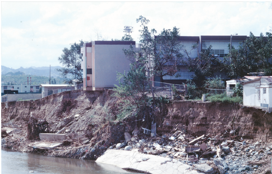
Figure F-3 This school in Puerto Rico was undermined by riverine erosion during Hurricane Georges in September 1998 (FEMA, 1999).
