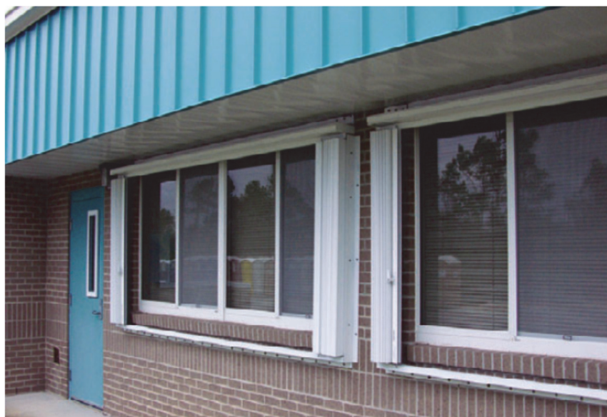
Figure H-15 This school was retrofitted with accordion shutters prior to a hurricane. The shutters successfully protected the windows from wind-borne debris during 2004 Hurricane Ivan (FEMA, 2010a).
