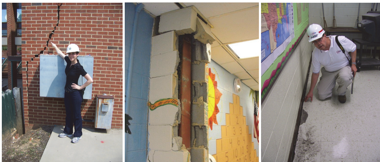
Figure 5-1 Photos documenting earthquake damage to school buildings. (Photo source: Michael Mahoney, FEMA)
