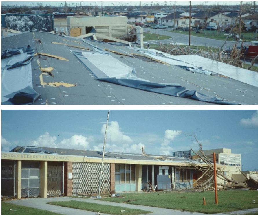
Figure H-12 Damage in a school in Florida during Hurricane Andrew in 1992. Several windows in this school were broken by wind-borne debris, and a large portion of the roof membrane blew off. Resulting interior water damage precluded quick resumption of school. (Photo source: Thomas Smith)
