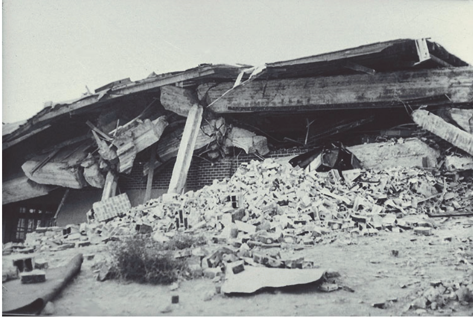
Figure E-5 Collapse of a portion of a concrete school in the Helena, Montana earthquake of 1935 (NISEE, 1935).
