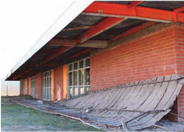
(a) Collapse of exterior soffit (i.e., exterior ceiling) at Jefferson Elementary School in the 2010 Baja, California earthquake. Soffit is made of plaster and is essentially the same weight as one inch of concrete.
