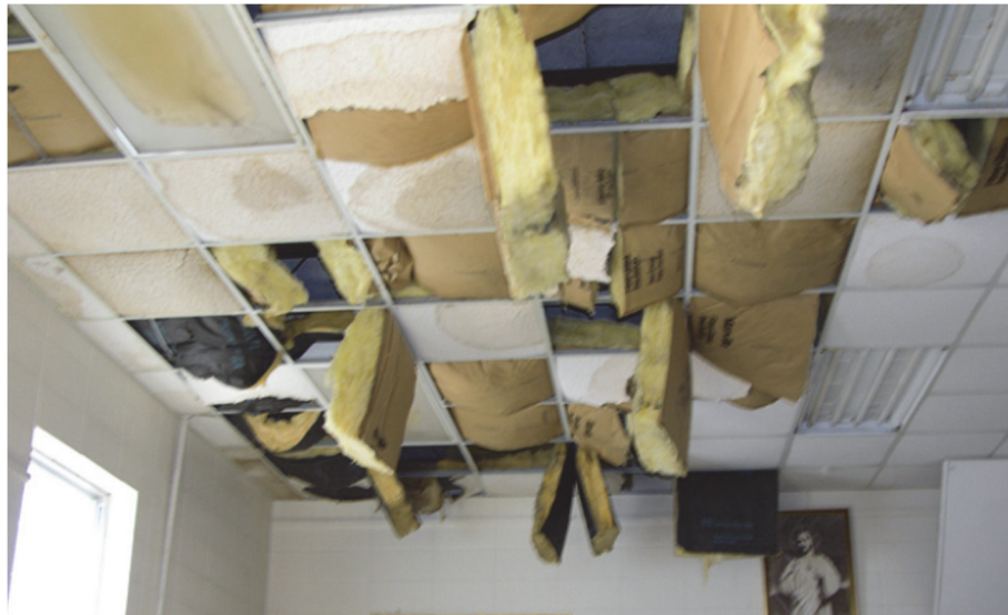
Figure H-4 Damage to school ceiling in Mississippi during 2005 Hurricane Katrina (FEMA, 2006b).
