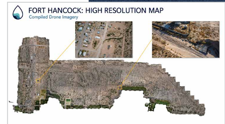
A high resolution map of Fort Hancock, Texas, created using compiled drone imagery. The inset images show arroyos that have the potential to flood. Source: Institute for a Disaster Resilient Texas.
