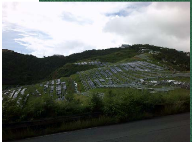
A solar farm destroyed by Hurricane Maria. © Hans Louis-Charles, 2017
