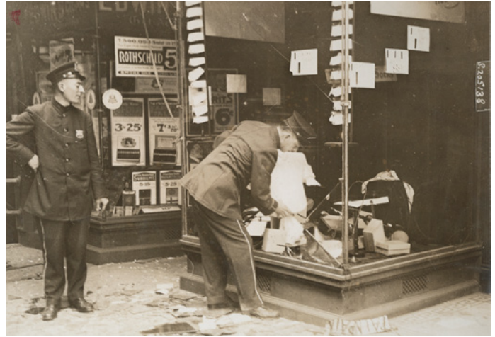
Shop on Warren Street guarded by two police men. This is one of hundred of shops in Lower New York City which had its windows shattered by the explosion of a carload of dynamite and 100 carloads of ammunition and shrapnel for the entente Allies. Policemen were placed on guard to prevent looting. © National Archives, 1916
