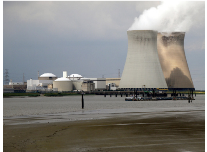
Doel, nuclear reactor © Torsade de Pointes 2013
