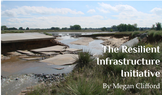
The Havana Pond Dam, City of Denver, Colorado breached and failed on Thursday, Sept. 12, 2013 © USFWS Mountain-Prairie 2013
