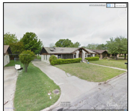
Image 1. Selected Levels of Damage
