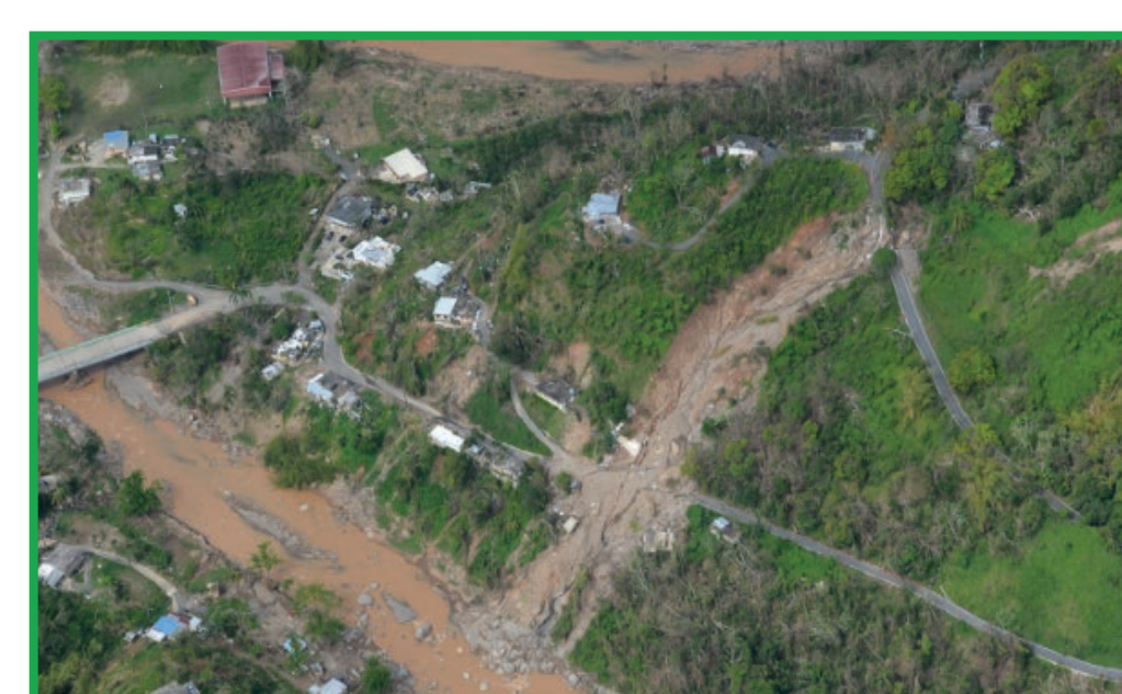
Figure 2. Landslide along PR-4131 in the municipality of Lares, Puerto Rico (Civil Air Patrol, 2017).
