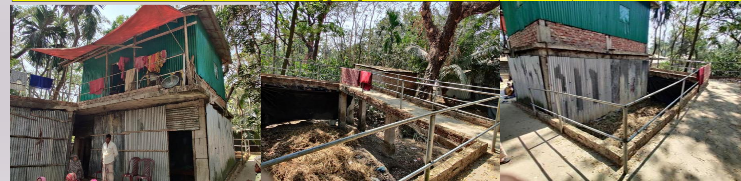
Photo: NGO-supported construction of disability-inclusive housing using indigenous resources and local knowledge to enhance accessibility, safety, and disaster resilience for households with persons with disabilities.
