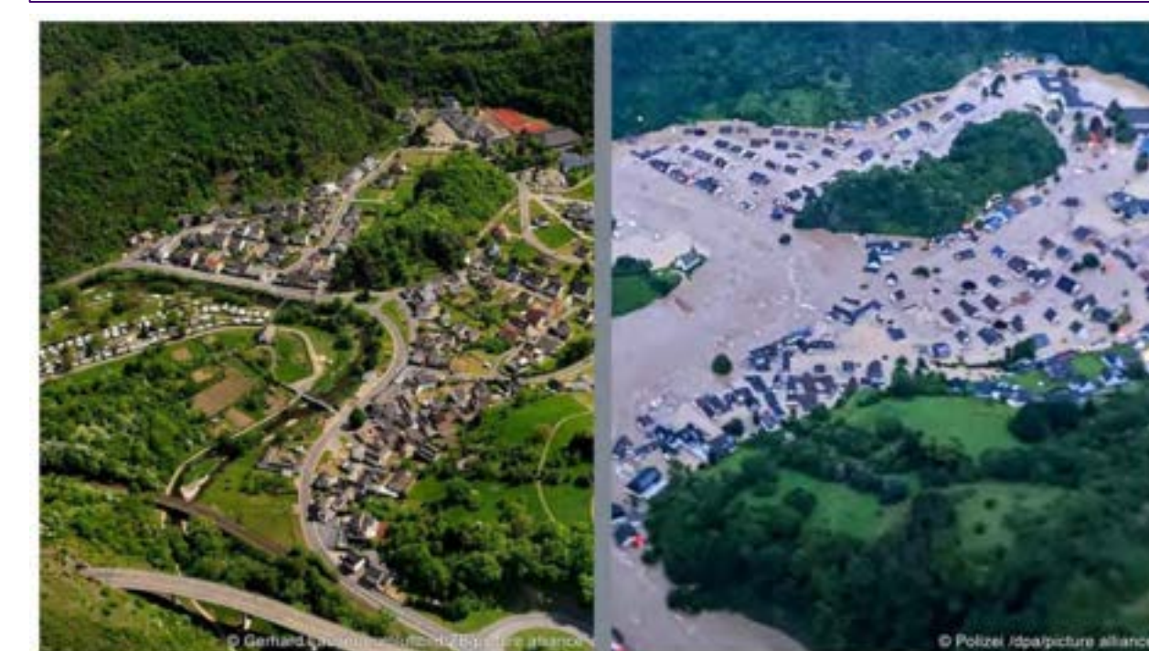
Pre-flood 2021 (Left) GEER Team August 2021 (Right)
