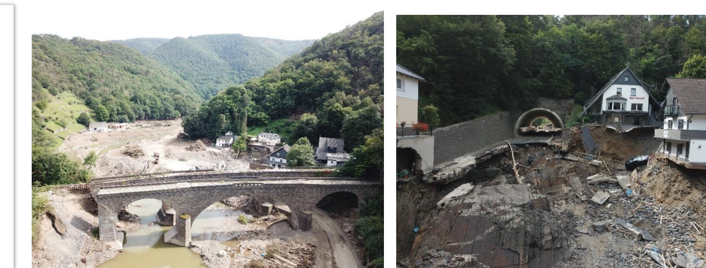
Figure 3. Altenahr's AM Tunnel (a) damaged bridges, water treatment facility, railway, and roadway; (b) damaged buildings, roadway, and tunnel; credit: GEER Team, August 2021
