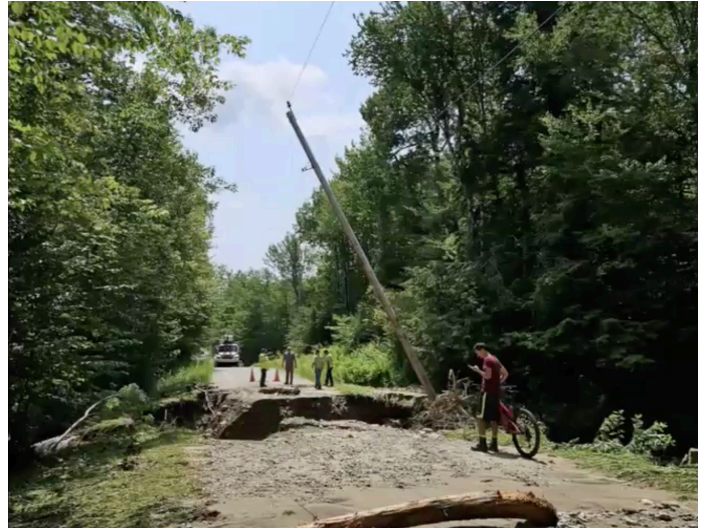
A normally small stream surged with water during the flood, eroding all roadway material around a culvert and creating a 12-foot crevasse that made the road impassable. Photo credit: Tim Banker, 2023.
