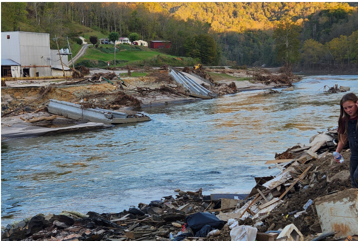
Hurricane Helene damage in Green Mountain, North Carolina, October 2024.
