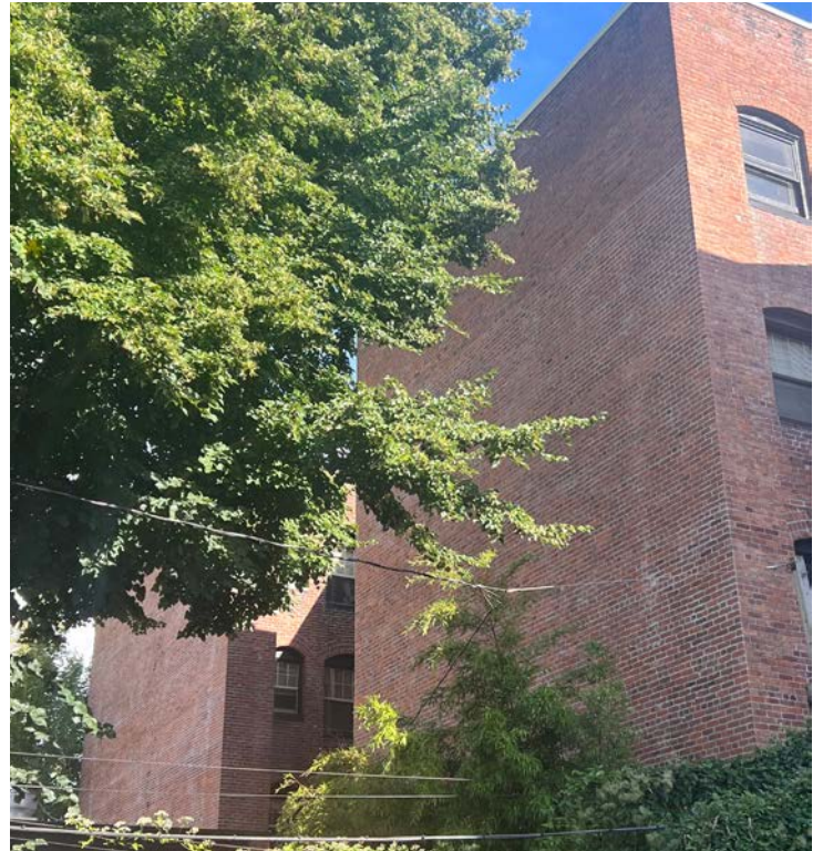
Example of an unreinforced masonry apartment
