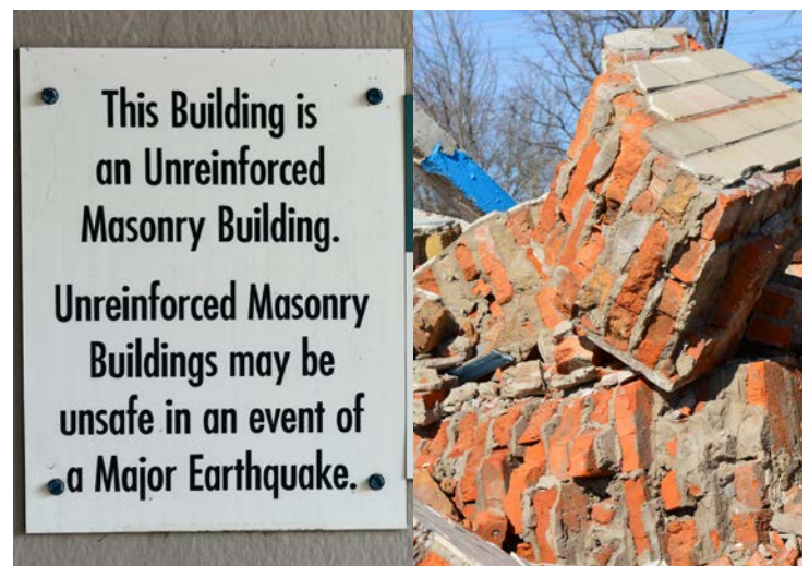
Image 1: Placard announcing unreinforced masonry building Image 2: A destroyed brick wall after an earthquake.
