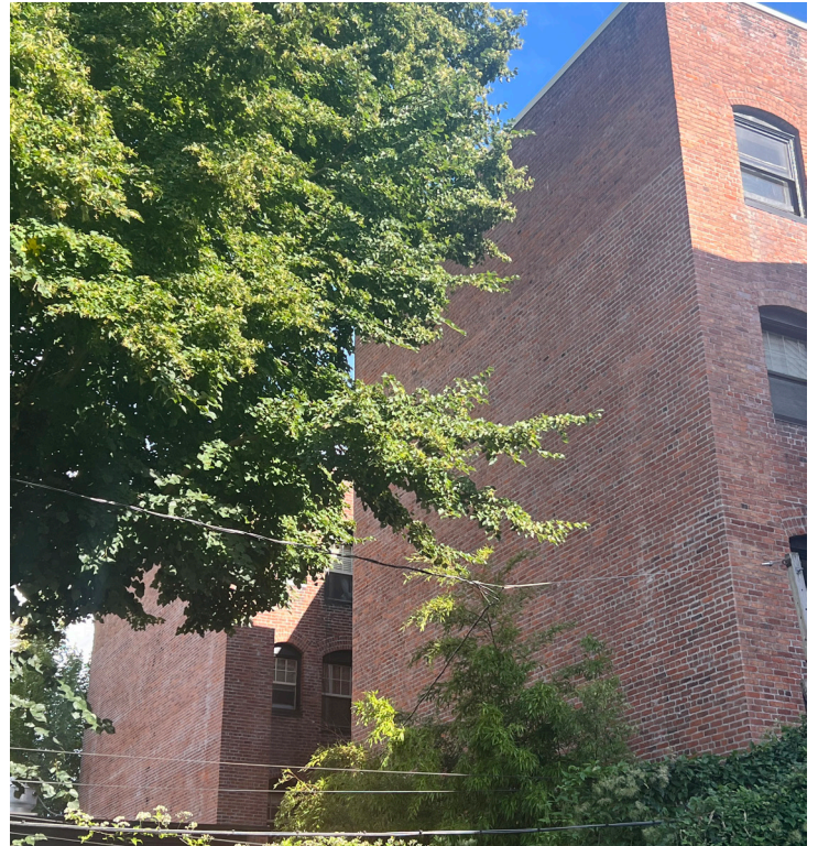
An unreinforced masonry apartment building in Portland, OR. Photo credit: Sarah Mercurio, August 30, 2023.
