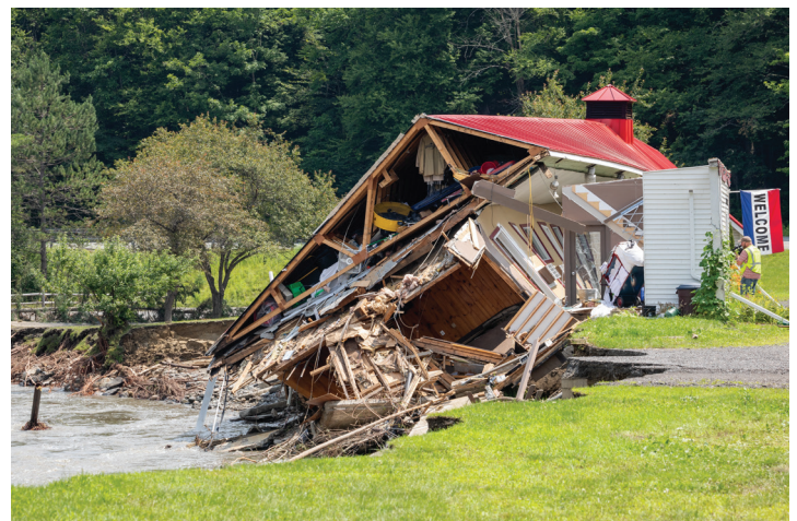
July 12, 2023: Flooding destroyed a motel on the Lamoille River in Hardwick, Vermont. Photo Credit: Mike Hardiman, Shutterstock.
