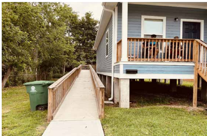
Elevated pier and beam home with ramp. Photo credit: Ivis García, Houston, Texas, March 2024.
