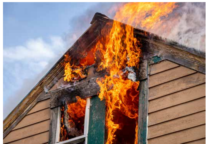
Fully engulfed structure fire
